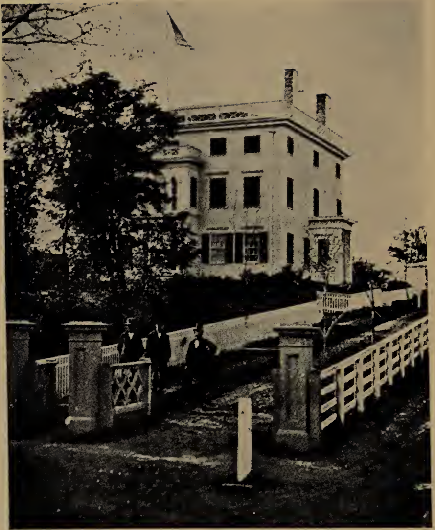
Caleb Cushing's Home High Street, Newburyport
